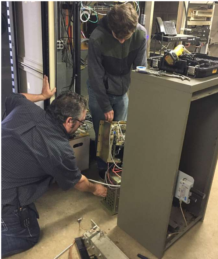
Robert KC8GPD and Skyler KGØSKY moving the 449.625 GE Master II out of the old rack
