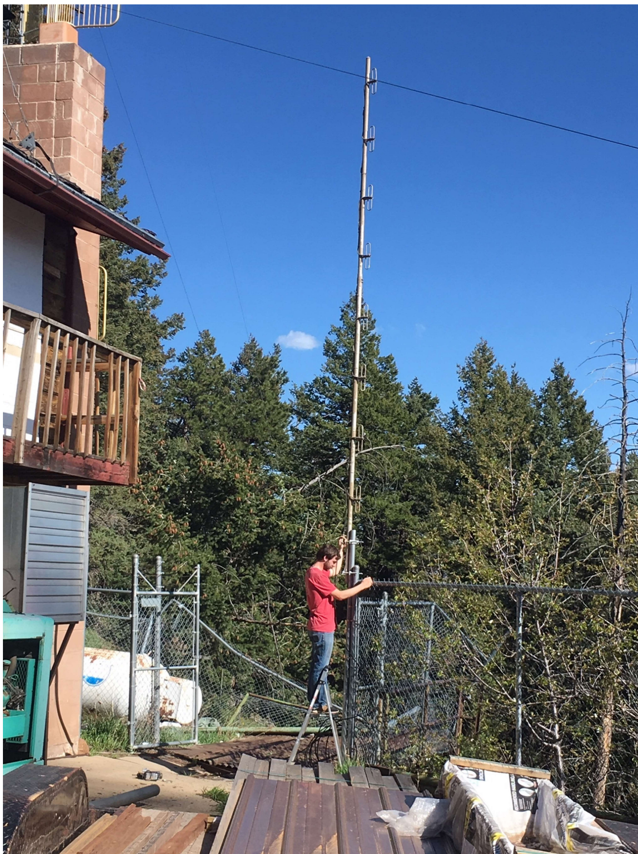
Skyler putting the sealant on the coax connection of the temporary testing standby antenna
