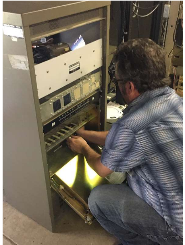
Robert KC8GPD and Skyler KGØSKY moving the 449.625 GE Master II out of the old rack
