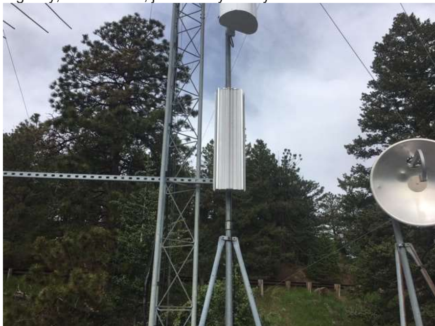
The link radio panel antenna above and #1 in the pic below
