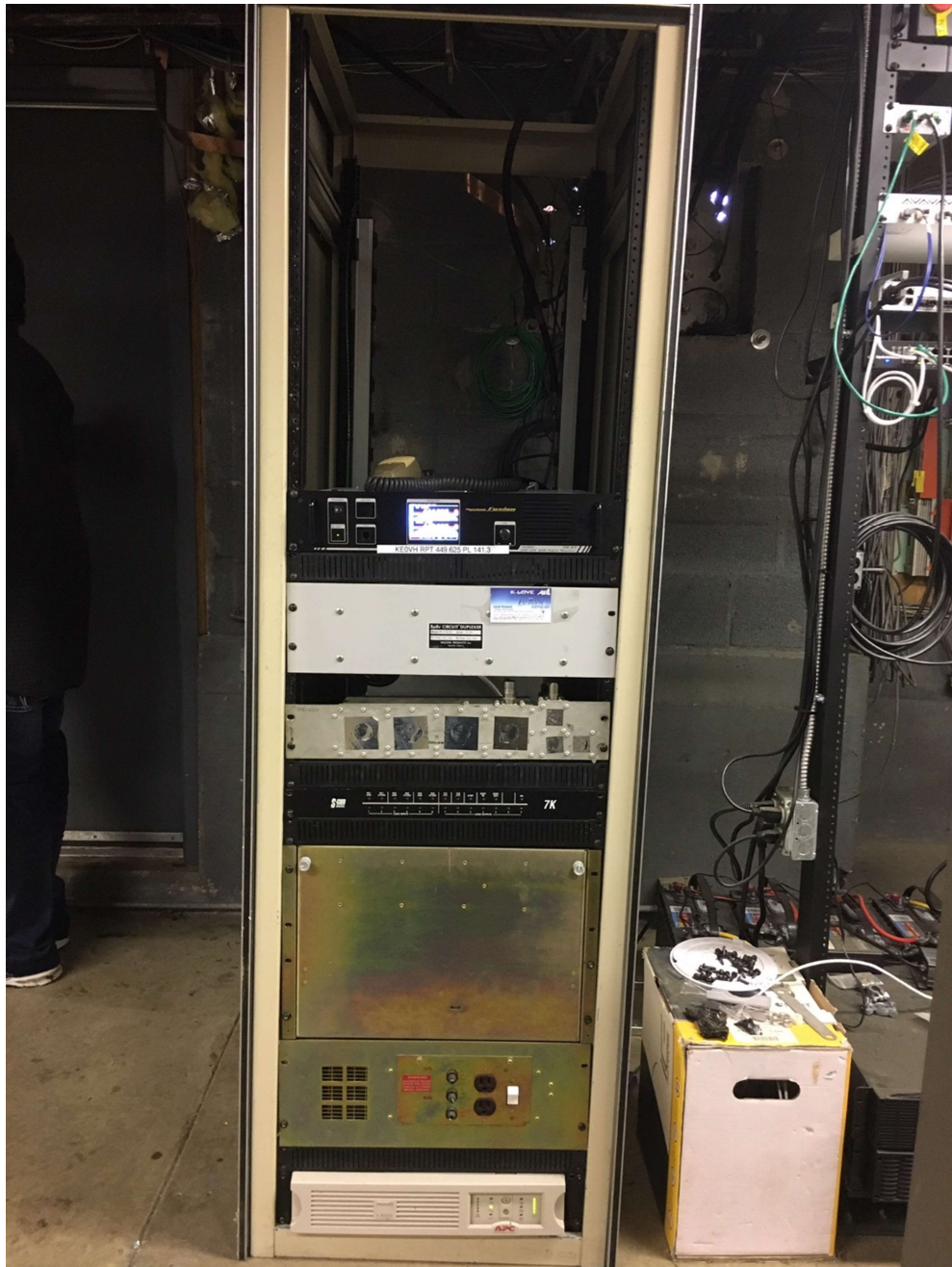
The new rack and home of 449.625 NOW KEØVH/RPT with the old GE Master II, S-Com controller, and the NEW FUSION REPEATER all setup and operating on air.
