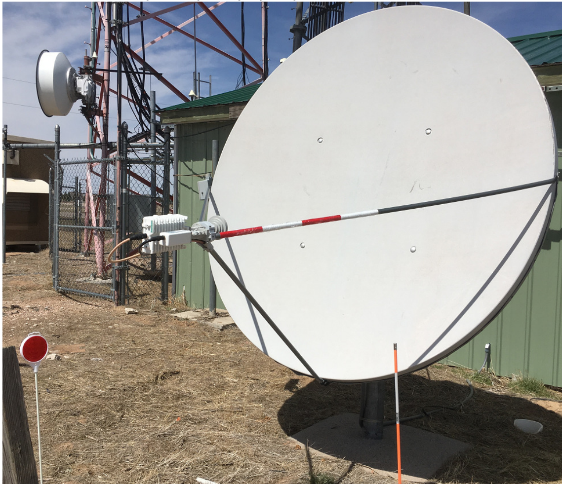
Repaired, cross-poled, and note the reflectors for future reference! ☺
