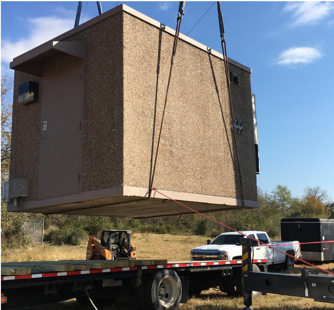
The building being lifted off the transport. Note the lines on the flat building bottom!
