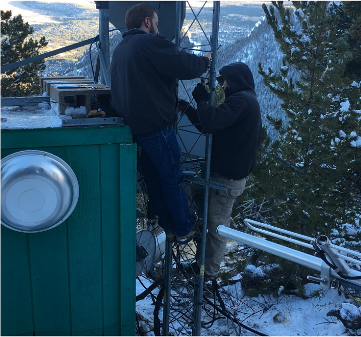
Kris and Eric working at the base of the temp tower, attaching it to a 5 foot section already in the ground, and Adam attaching our antenna
