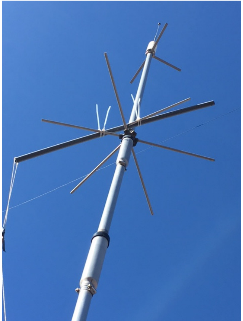
Side view of the original mount and the wind broken spar and “spider”
